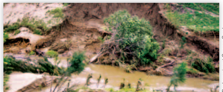
Bank erosion at Carron Creek, SEQ Catchments
